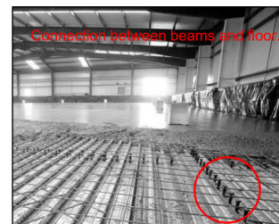
Welded studs: very difficult to detach beams from slab.
