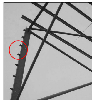
Cleats to support secondary steelwork. Can be removed.
