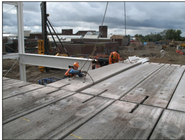
Precast units with floor bracing system
