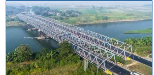
Long-Span Truss Bridges
