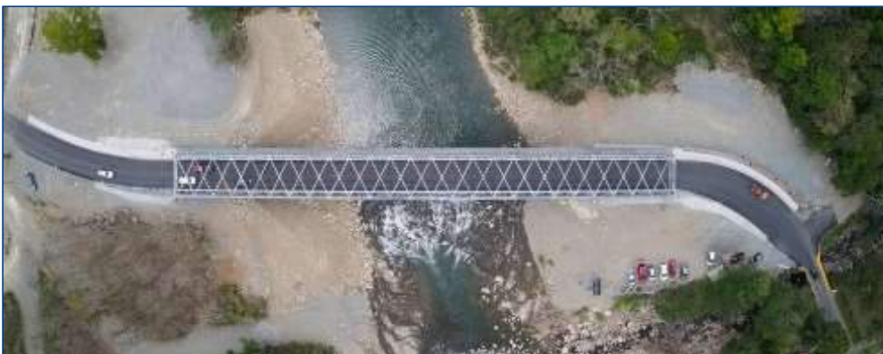
Long-span modular steel bridge Puente General Viejo in Costa Rica
