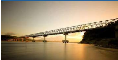
Calaba Bridge in the Philippines
