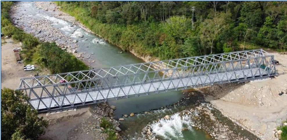
Long-span modular steel bridge Puente General Viejo in Costa Rica
