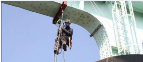
Installation services in Central Europe
