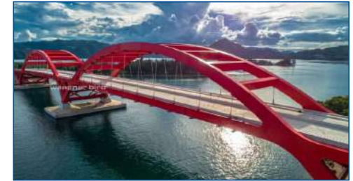
Youtefa Box Arch Bridge
