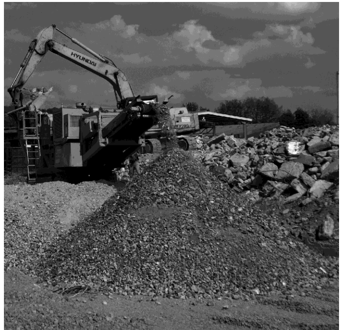
Figure 3. Gravel of concrete after recycling the waste on-site.
