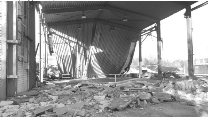
Figure 6. View of the hall with removed facade.
