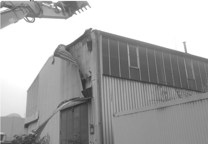
Figure 5. Removing of steel and capsuled insulation by excavator work.
