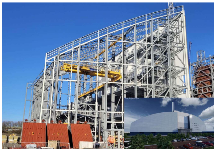
© Billington Structures Ltd , © Weedon Architects
