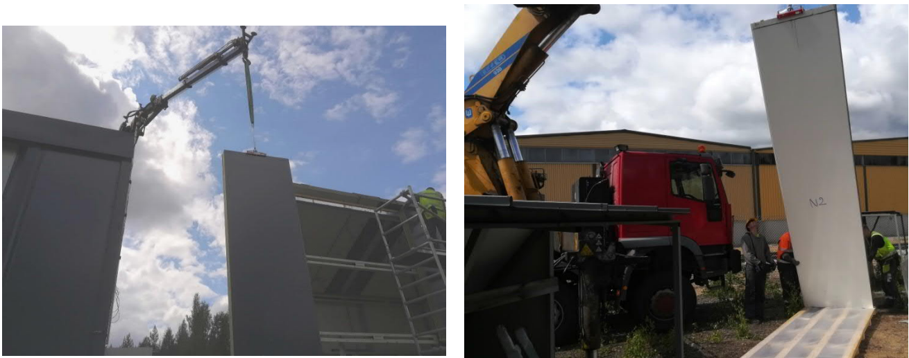
Figure 18 Dismounting of panels with crane.
