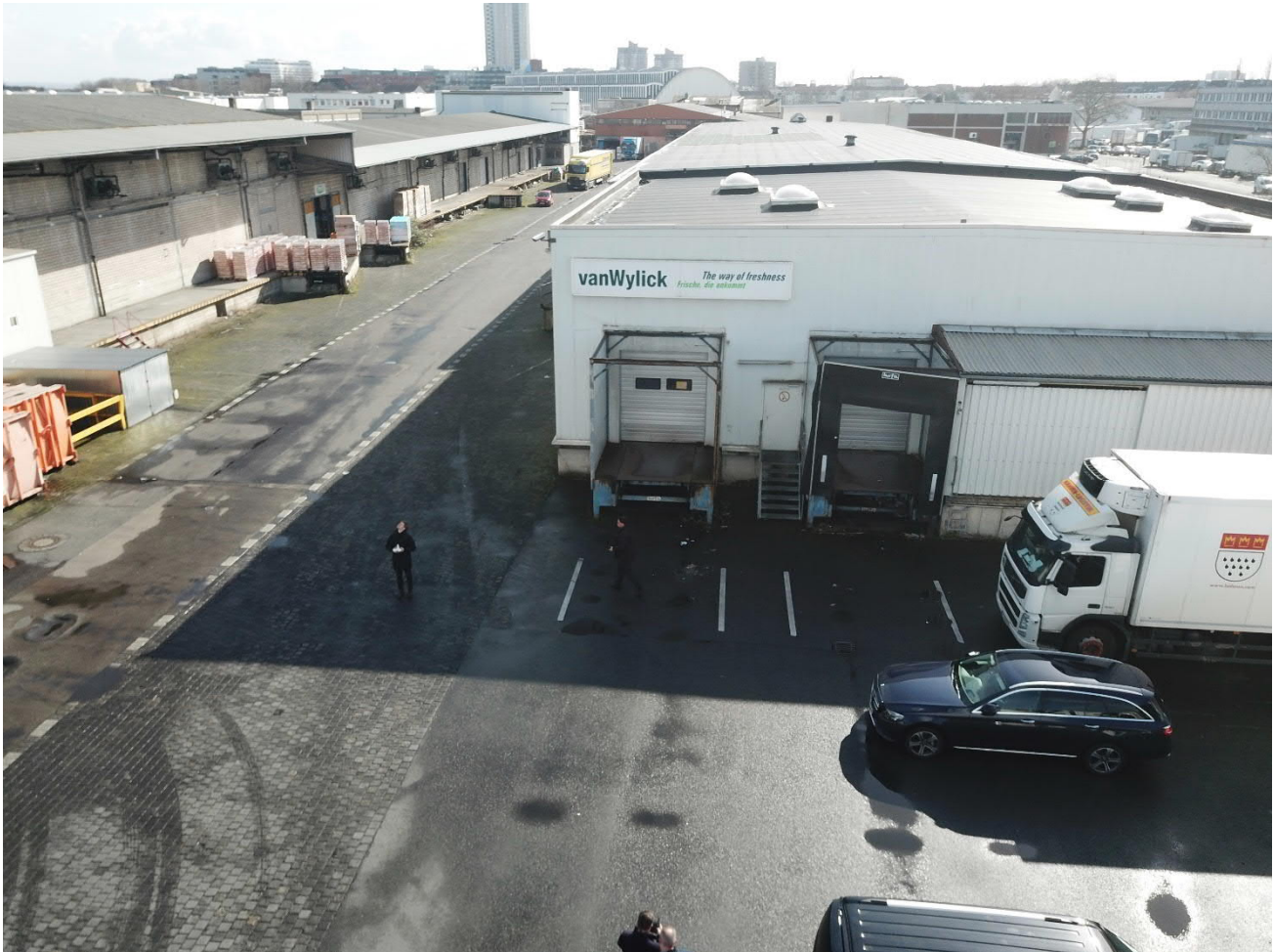
Figure 2 View through the market area with the single storey hall to be deconstructed on the right.
