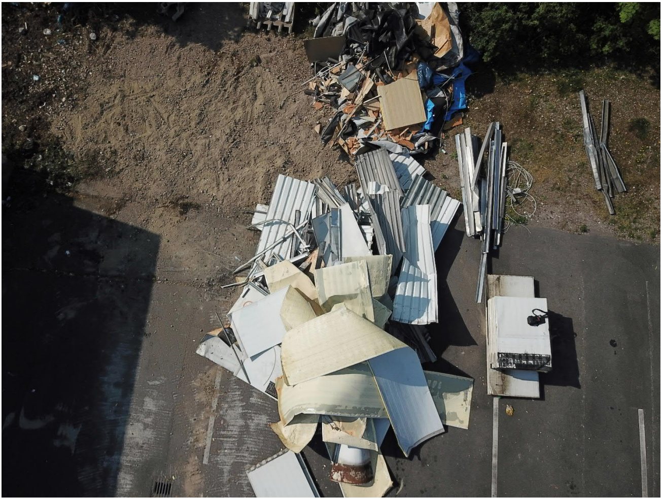
Figure 17: Sorted waste for recycling. Mixture of trapezoidal sheets and sheets from sandwich elements.
