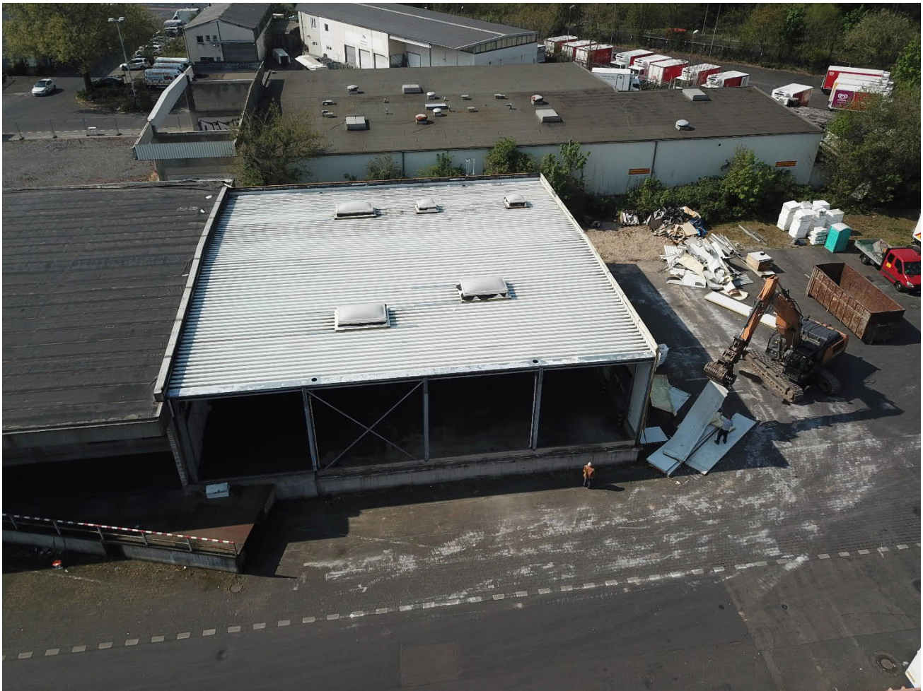
Figure 13: SSB with removed roof insulation and removed walls of sandwich elements. On the right, an excavator is starting to separate the metal sheets from the inner insulation of the sandwich elements.
