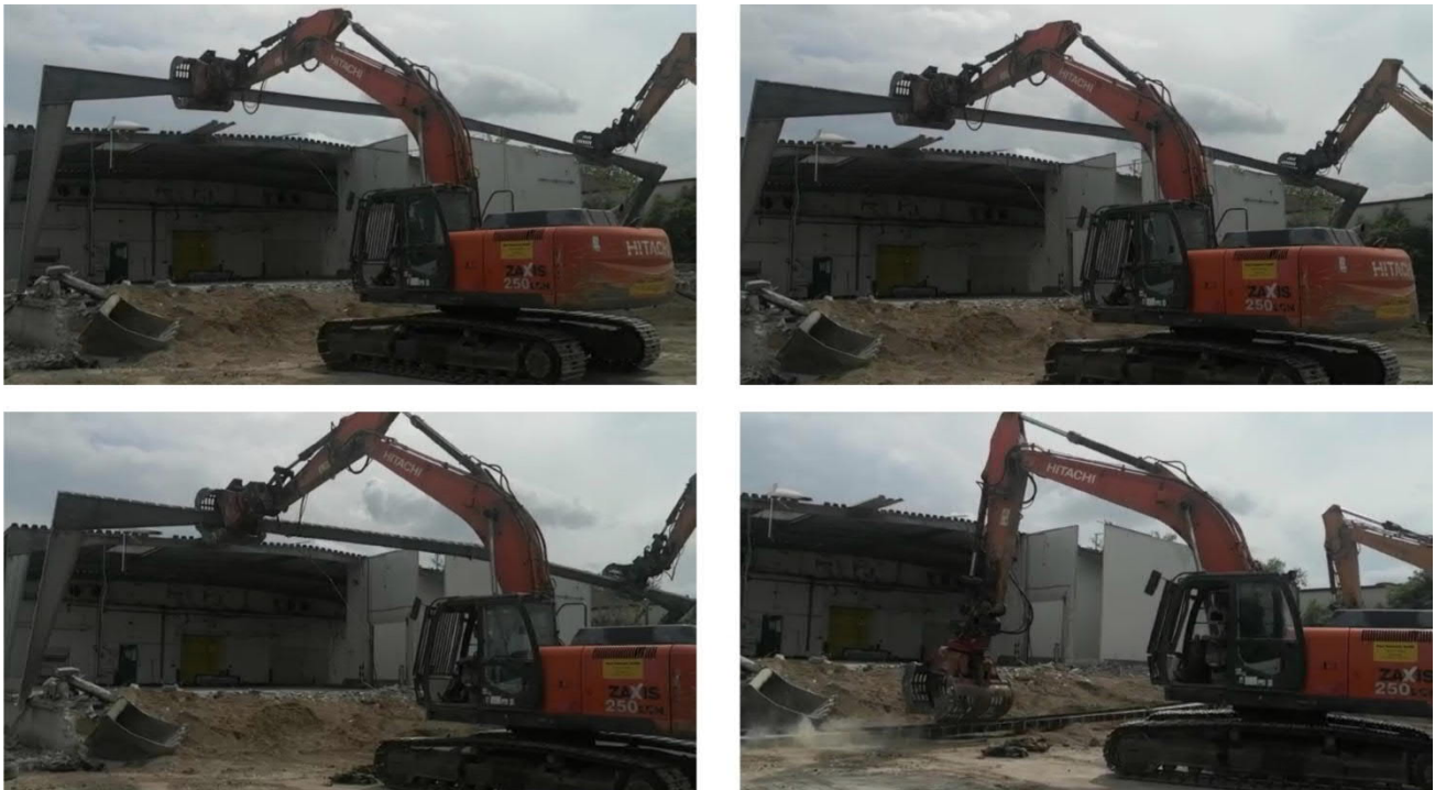
Figure 21: To avoid instabilities, two excavators carefully pull down the structure to the ground.
