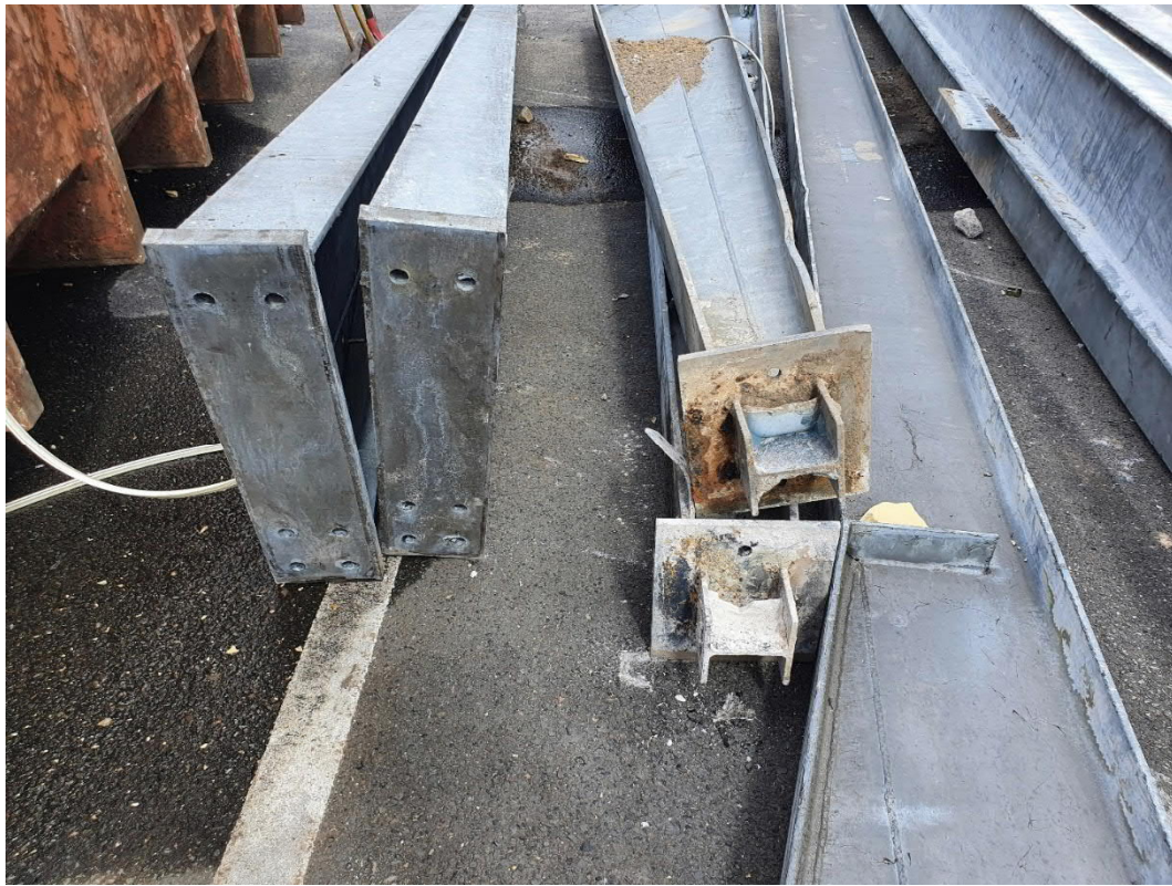
Figure 26: deconstructed parts of primary structure ready to be reused.
