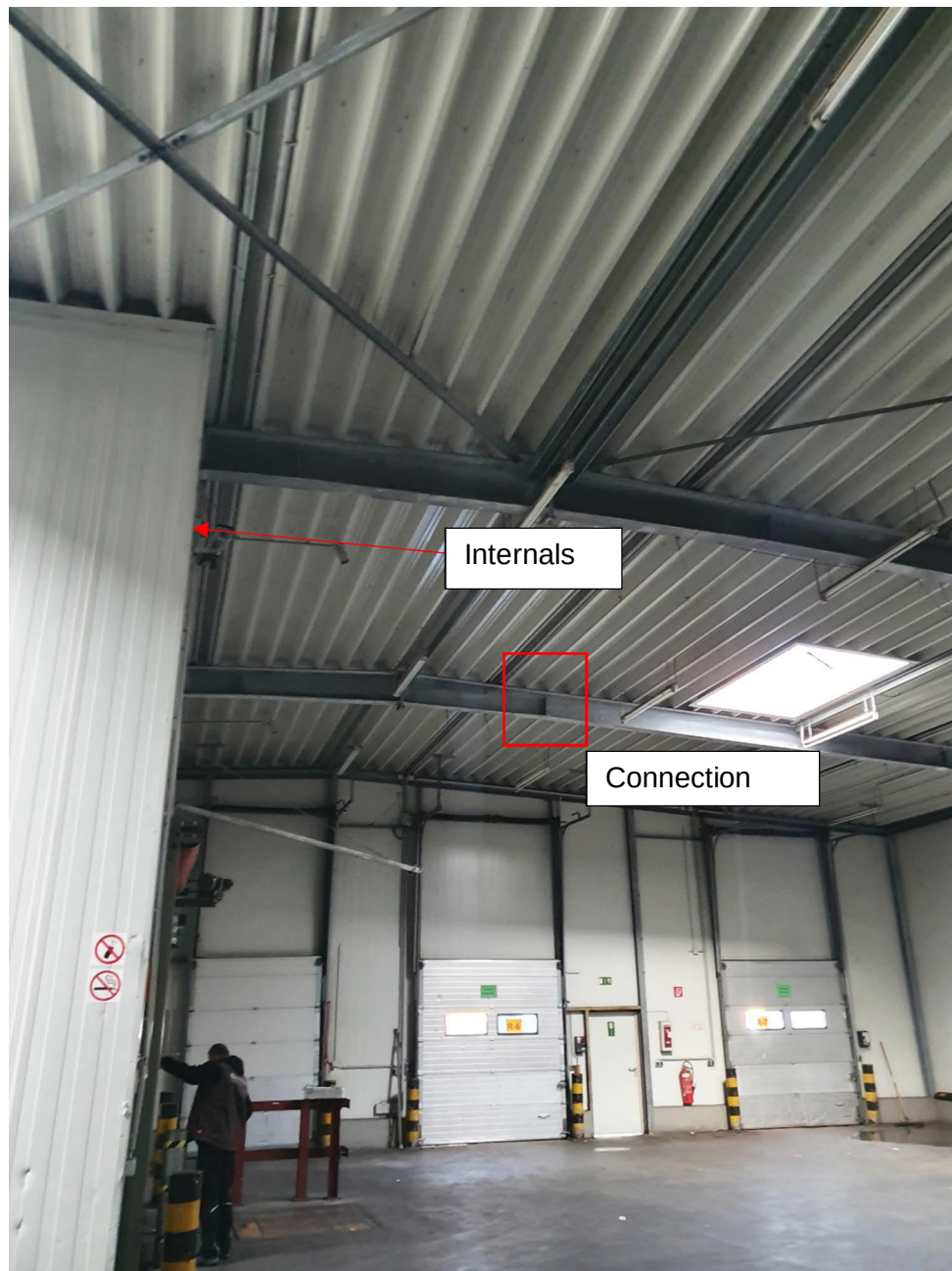
Figure 6: Inside there are 2 rooms. The walls between those rooms were made of cladding walls.
