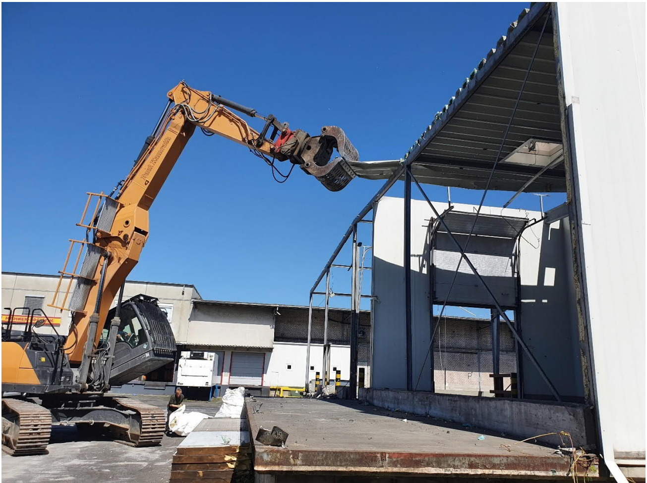
Figure 16: Dismantling old trapezoidal sheets just before deconstruction of structure.
