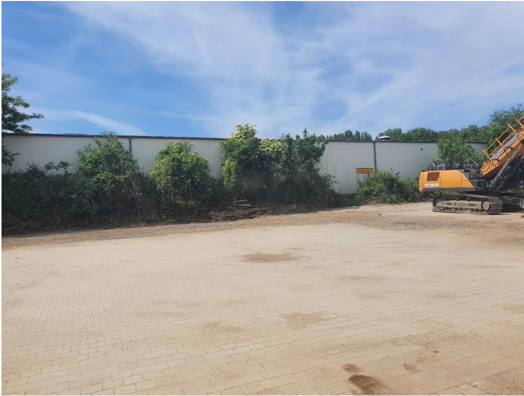
Figure 25: Area of the SSB afterwards. The site is cleaned up.
