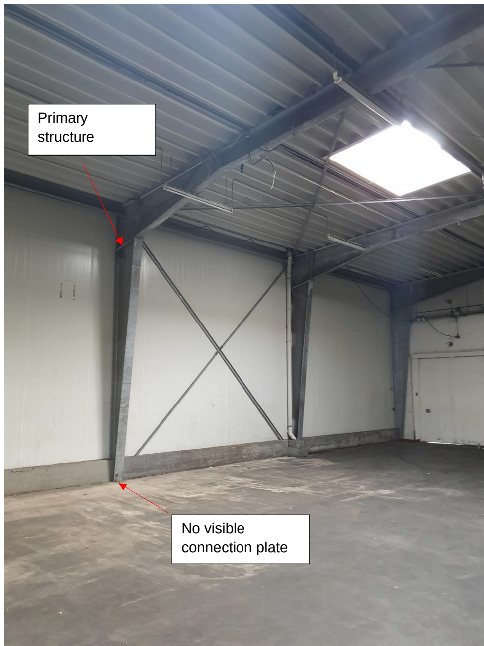
Figure 4: Steel structure: The primary structure is made of 4 steel frames. There is no visible connection plate on the ground. Obviously, the columns are grouted with the concrete.
