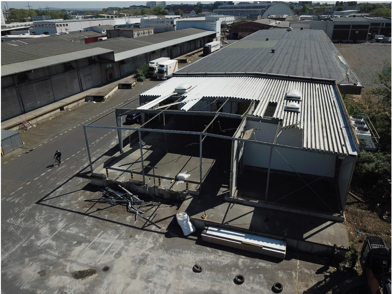
Figure 19: The hall during the process of dismantling just before deconstruction of the structure. The trapezoidal sheets are being removed by 50%. Only the structure is remaining. After the removal of the trapezoidal sheets all remaining steel parts are considered for reuse.
