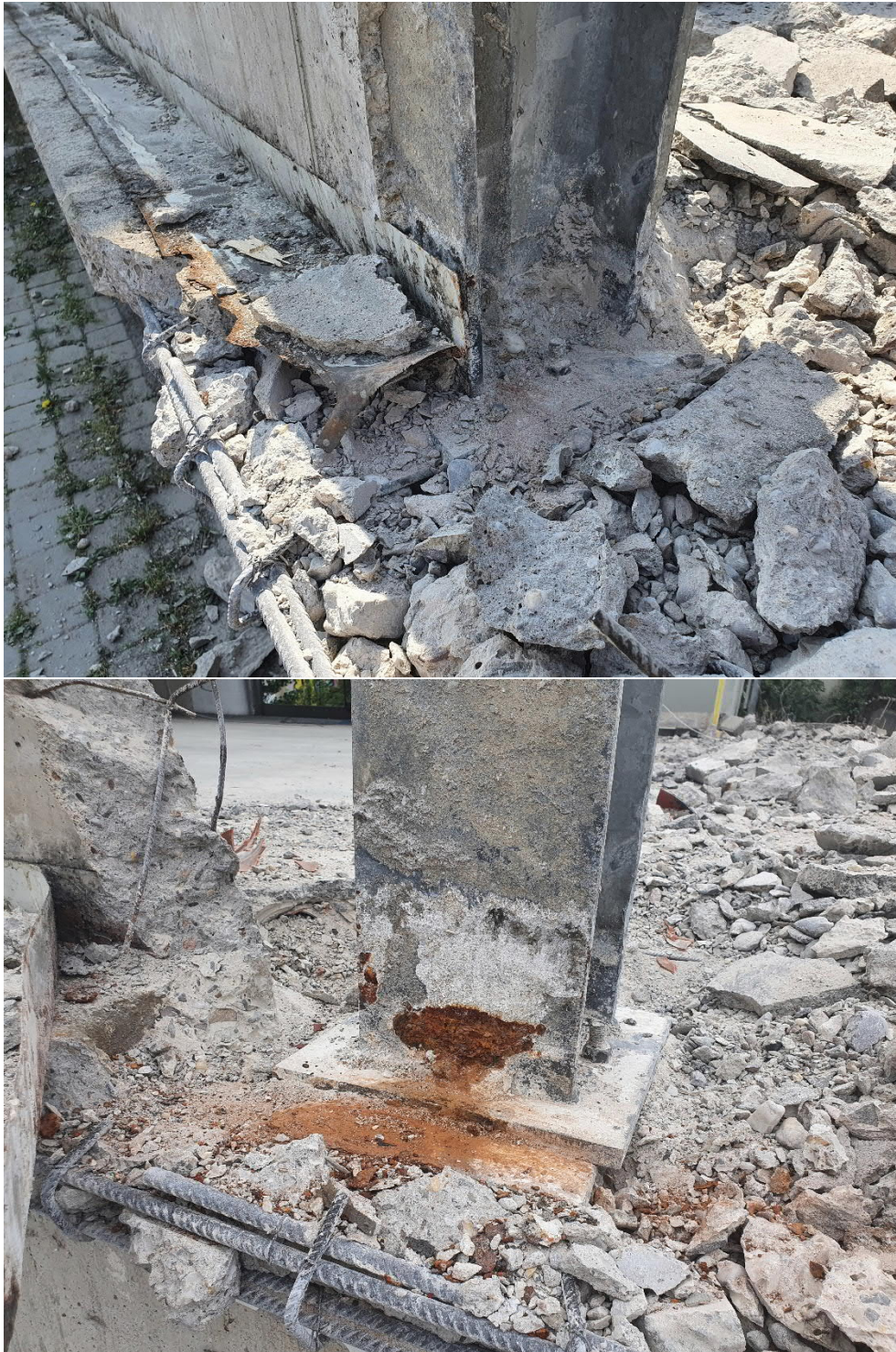
Figure 22: Removing concrete at jointing of steel frames. The steel connections was shed below the floor plate directly on the fundaments. Afterwards the connections was shed into the concrete of the floor plate. To release this connection, the concrete was removed partly around the anchoring.
