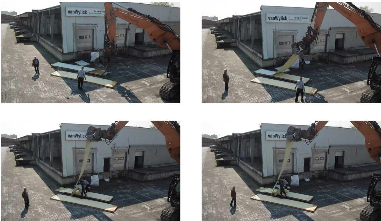
Figure 15: Separation of metal sheets by help of excavator and two workers
