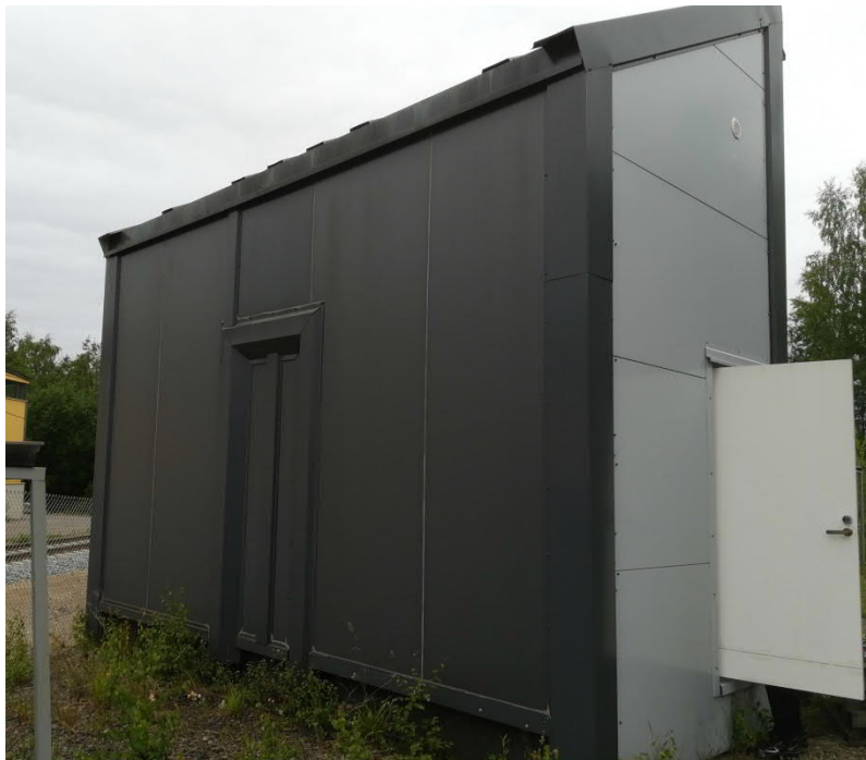
Figure 16 Test building from where sandwich panels were dismantled (South façade)
