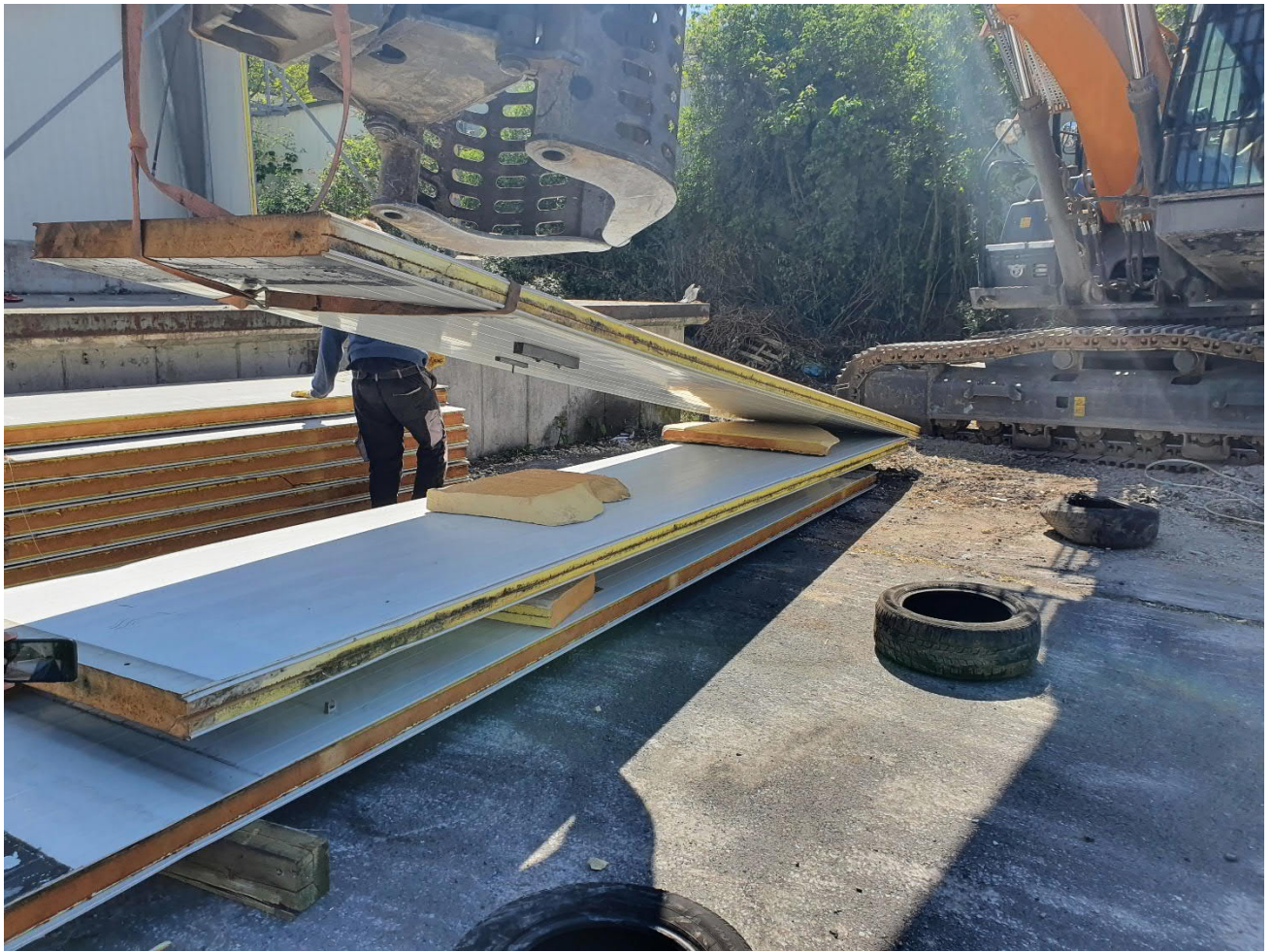
Figure 14: Dismantling of sandwich sheets. Testing of reusability. Technically, safe dismantling is possible by excavators. Reuse might not be recommended since the glue between metal and insulation is weathered. Besides, the metal sheets have many holes e.g. from attached lamps, signs and other inventory attached to the sheets.
