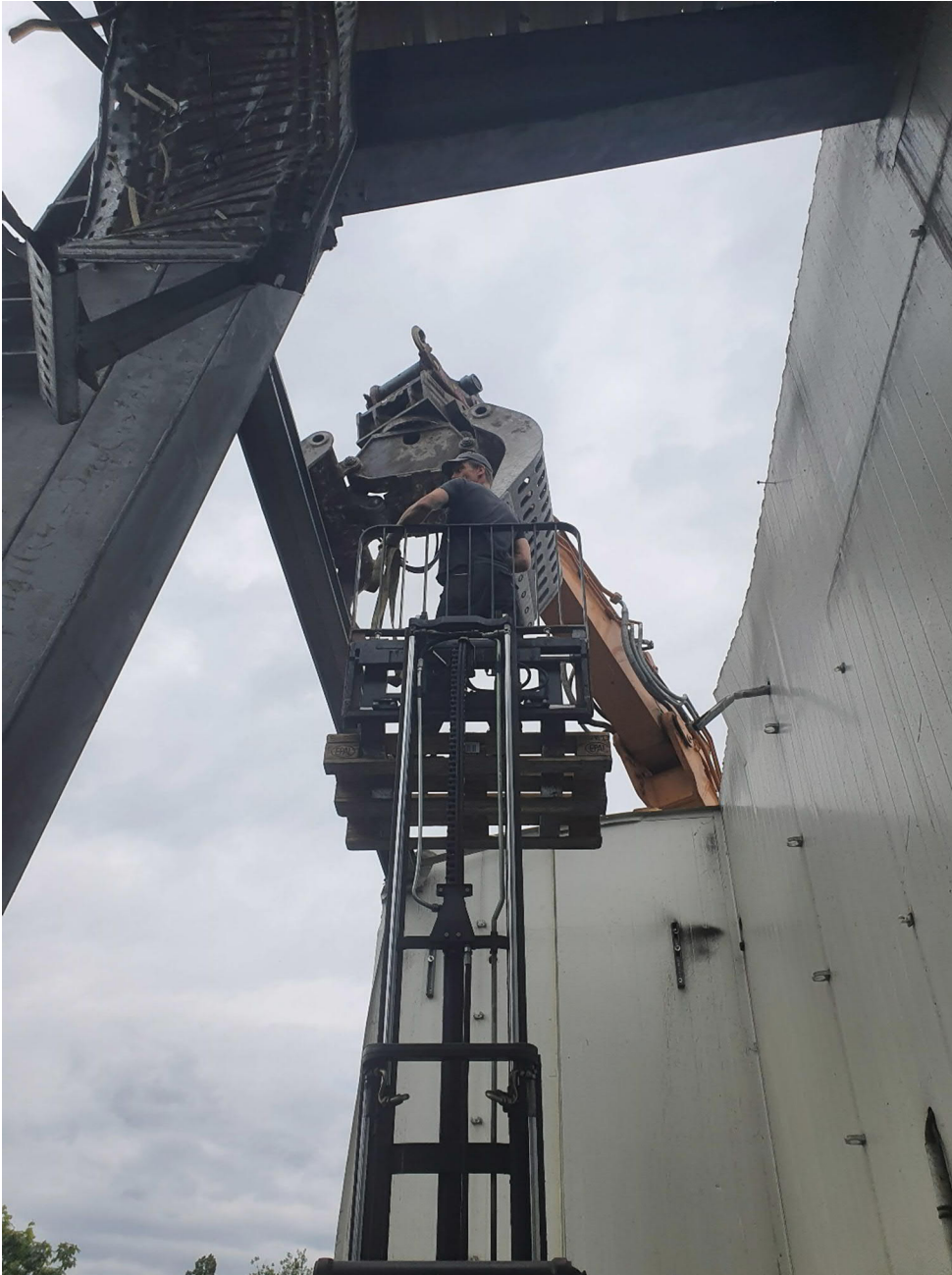
Figure 18: Dismantling of secondary structure. These parts are still too thin, that handling with an excavator only would result deformation. On the other hand, these parts are not tending to deform as long as dismantled manually. In opposite to the cladding, only five elements between each section are to dismantle.
