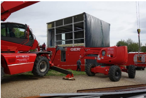
Figure 21 Dismantling Process of Sandwich-Demo-House
