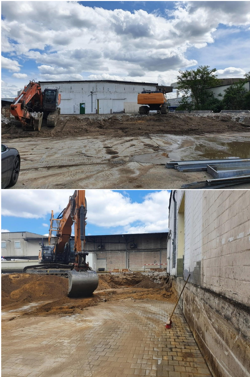
Figure 24: Demolition of concrete slab and removal of sand filling. Below the old pavement was recovered.
