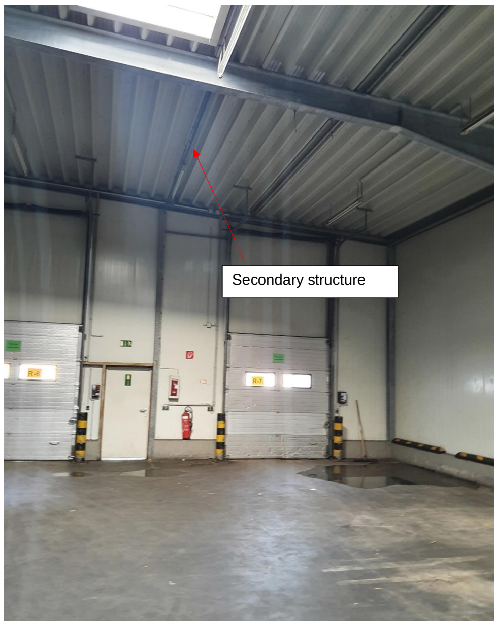
Figure 5: Between each of the frames smaller cold-formed steel beams as a secondary structure are visible. The connections are screwed.
