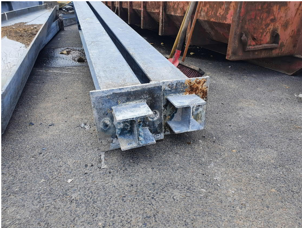
Figure 23: View from the downside of the connection. The plates were connected to the fundamentals and shed into the concrete of the ground floor plate.
