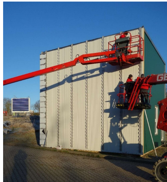
Figure 42 Installation of profiles with one-sided fixation
