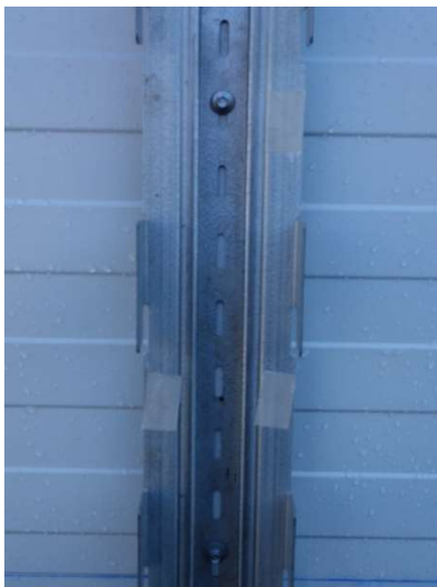
Figure 42 Installation of profiles with one-sided fixation
