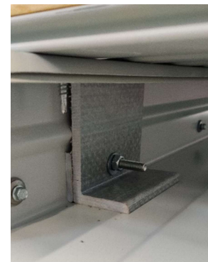
(b) Detail of liner tray web reinforcement
