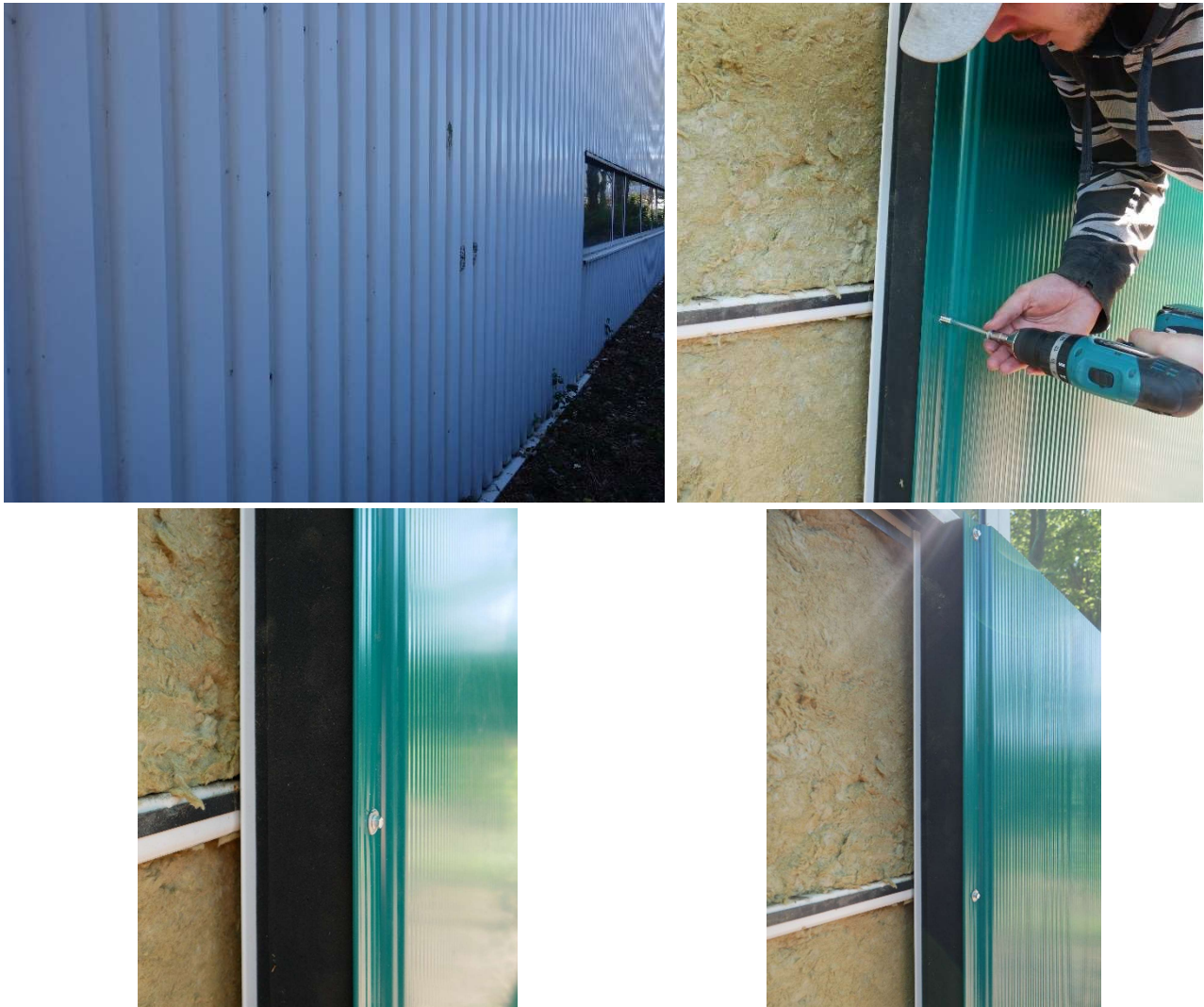
Figure 43 Installation of hybrid system
