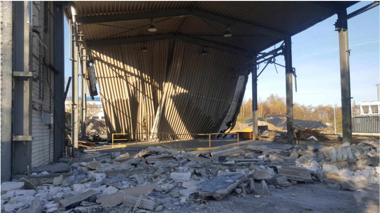
Figure 1.19 Partly demolished hall. At this stage all side walls were demolished and the insulation removed and structure was demolished using excavators
