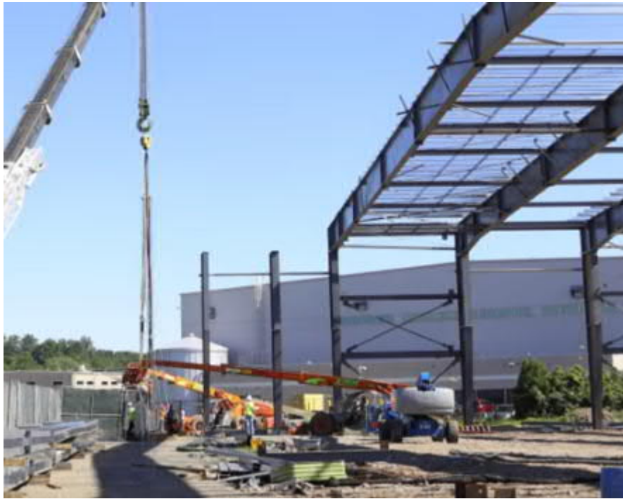
Figure 1.36 Isolated columns with out of plane restraint ready to be deconstructed
