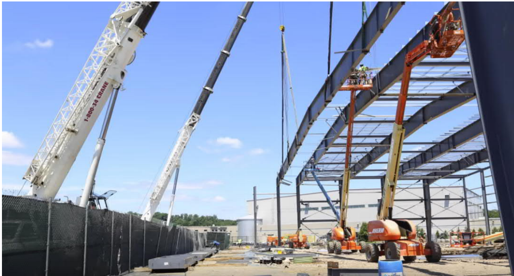
Figure 1.33 Rafters supported by mobile cranes during purlins installation/removal.
