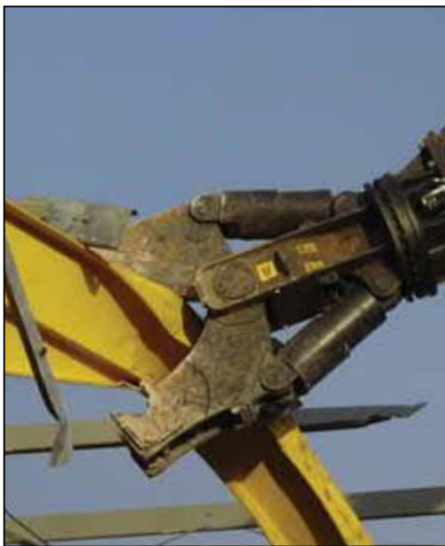
Figure 1.13 Steel shear attachment pulling-down and shearing a steel structure
