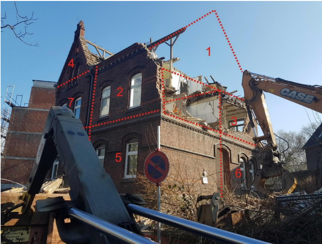
Figure 1.7 Demolition of a large brick house using the Room-by-Room method
