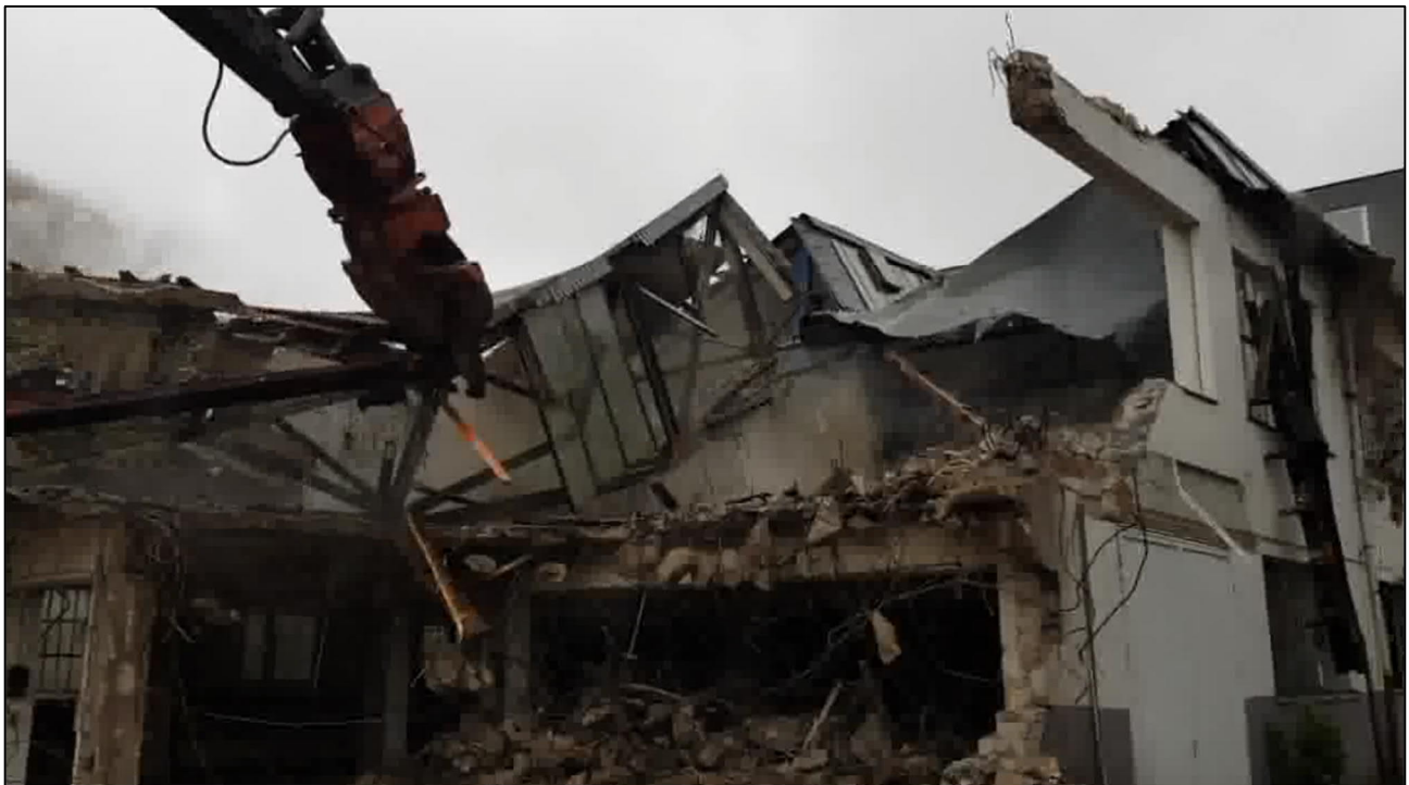
Figure 1.2 Modern demolition practice is generally a destructive technique without consideration of recovery of elements of the building for possible reuse
