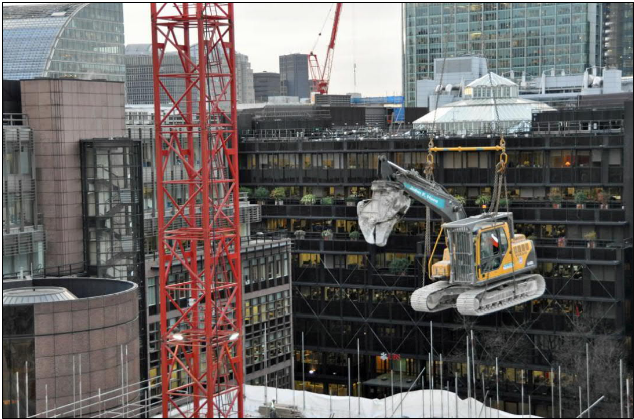
Figure 1.3 Hoisting an excavator using a tower crane for top-down demolition of a large multi-storey building in London
