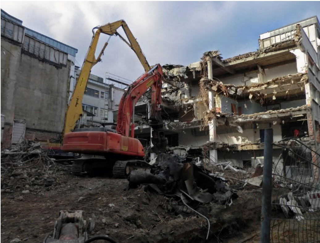
Figure 1.4 Typical top-down demolition of a concrete building using a high-reach excavator
