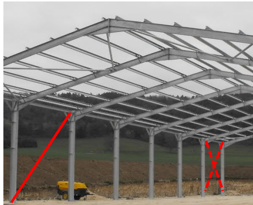
Figure 1.31 Examples of temporary bracings.
