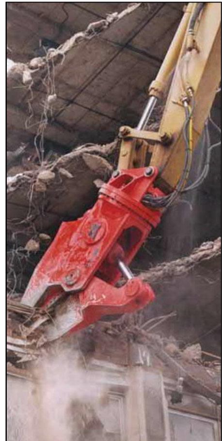
Figure 1.12 High-reach excavator demolishing a concrete structure (left). Rotating pulveriser (right)
