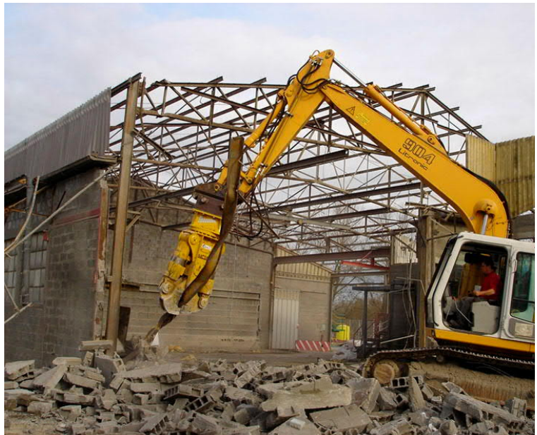
Figure 1.13 Steel shear attachment pulling-down and shearing a steel structure
