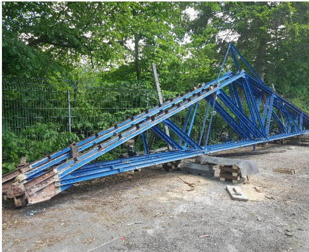
Figure 1.22 Images during the deconstruction project and the recovered roof trusses
