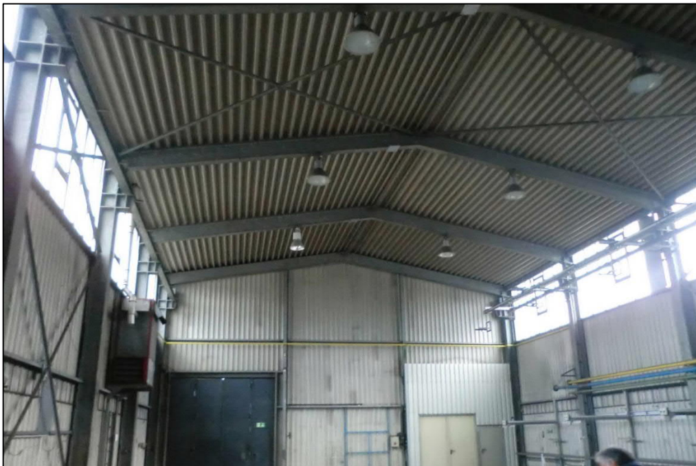
Figure 1.18 View inside the single-storey hall of 407m 2
