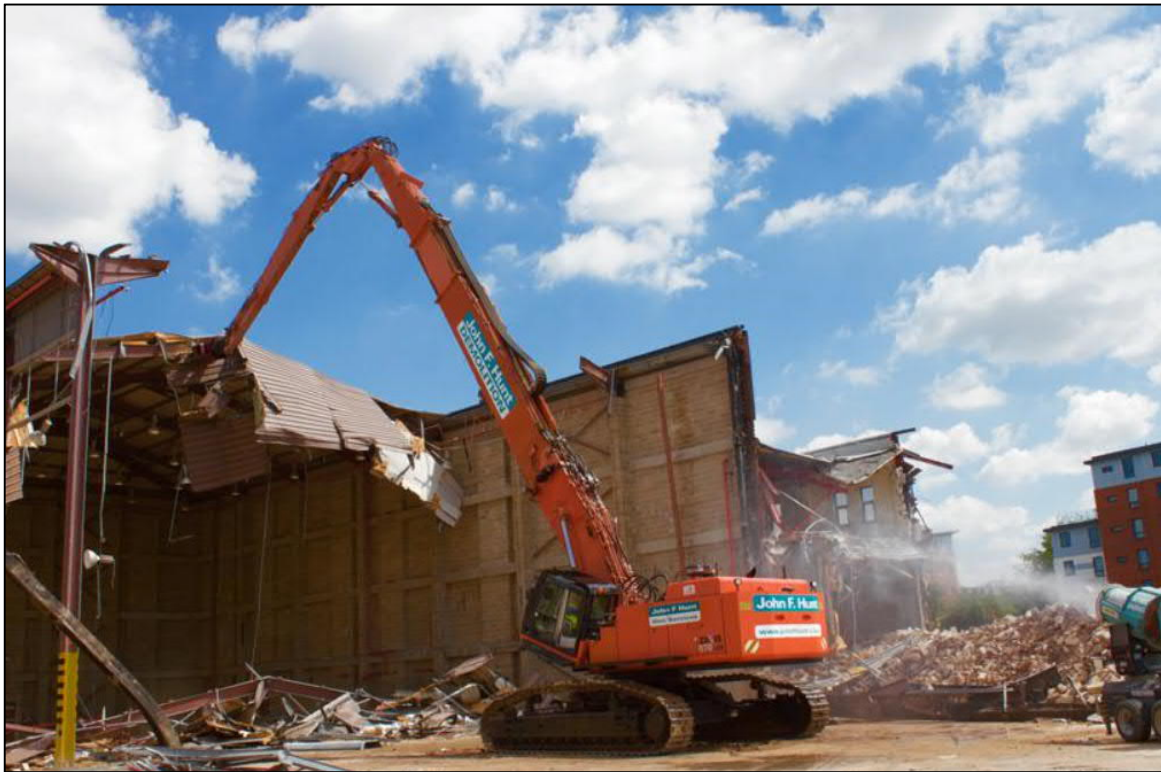
Figure 1.10 Excavator being used to demolish a low-rise steel-structure
