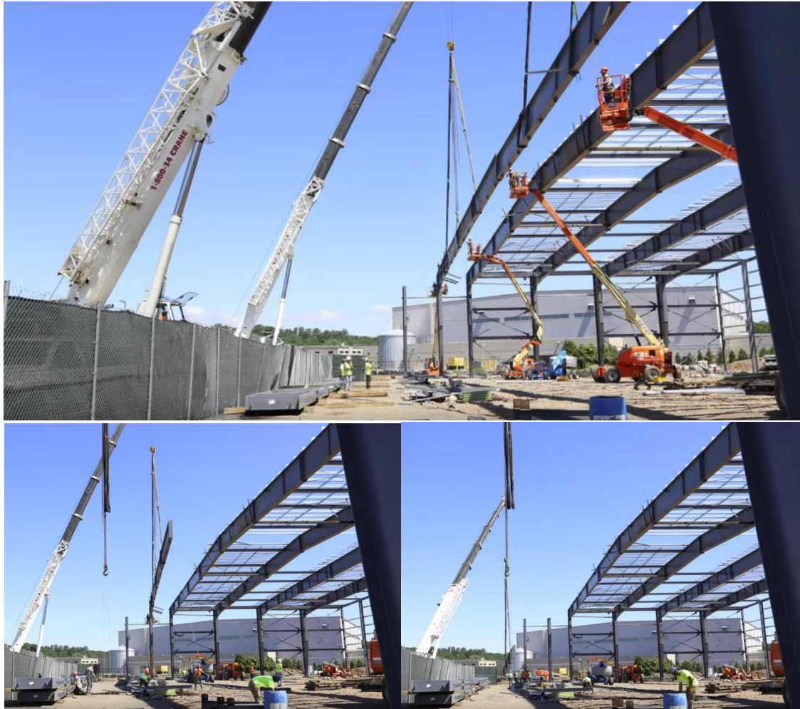
Figure 1.35 Erection/deconstruction of individual long span rafters
