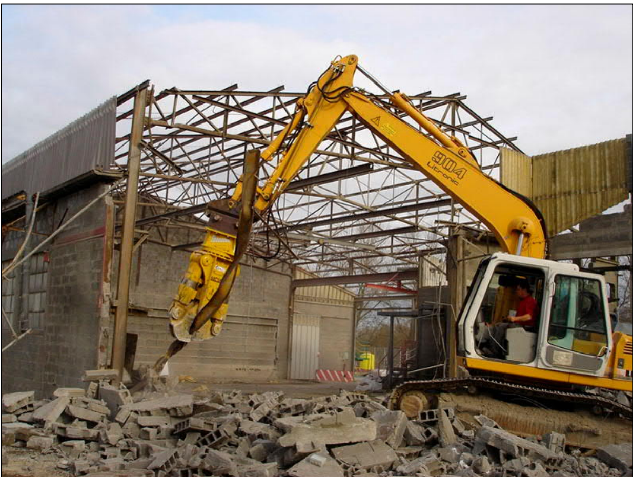
Figure 1.15 Excavator with hydraulic shear attachment to cut steel beams into manageable lengths
