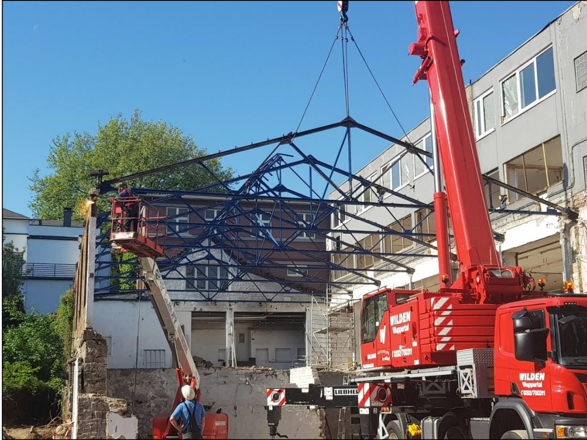
Figure 1.20 Deconstruction and reuse of steel roof structure
