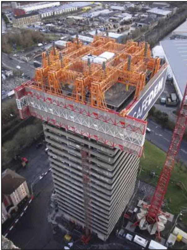
Figure 1.6 DESPE modular, top-down demolition system used to demolish an apartment building in Glasgow
