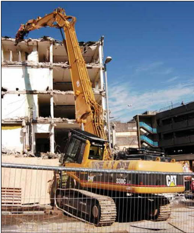
Figure 1.12 High-reach excavator demolishing a concrete structure (left). Rotating pulveriser (right)
