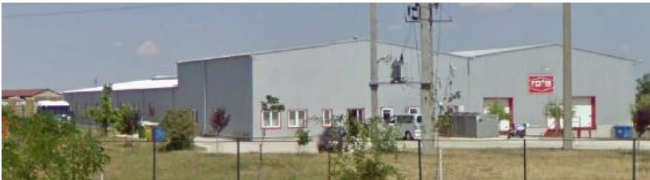
Fig. 2. Case-study steel building in Arad, Romania
