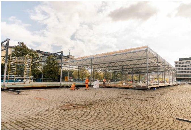
Picture 1 Deconstruction of steel frame hall in Hakaniemi, Finland
