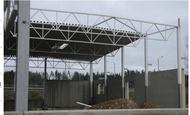
Erection of the steel frame in new location
