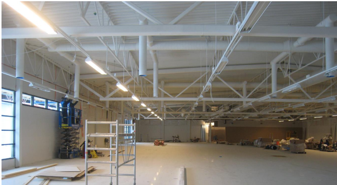
Internal view of the new building
