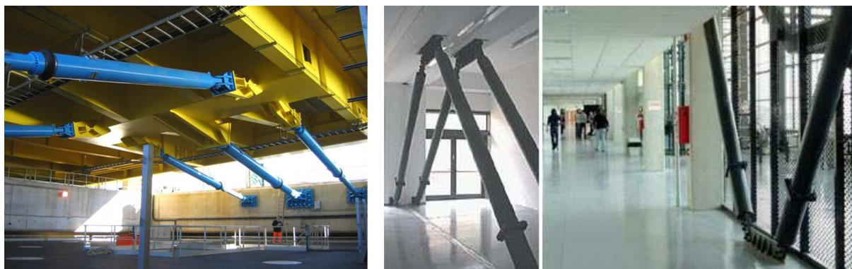
a) Viscous dampers applied in the Rion-Antirion Bridge (Greece) - (Courtesy: FIPMEC srl)
