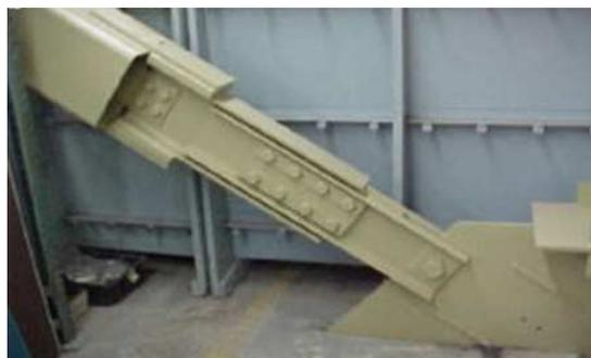
b) Pall devices installed in a single-diagonal brace at Boeing Commercial Airplane Factory Everett, USA - (Ref: Dr Pall)
