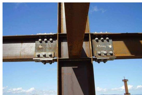
b) Sliding hinge joint with asymmetric friction dampers of the award-winning Te Puni Village of Wellington - [13]
