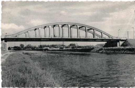
Pont Hasselt, Belgium, 1938
