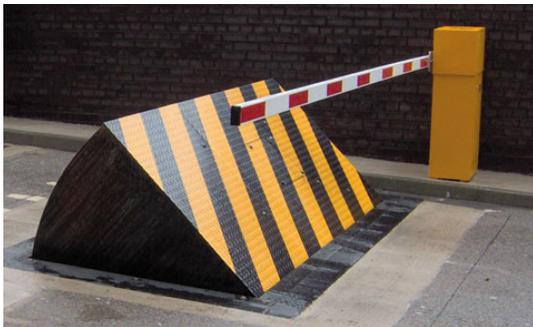
Figure 8. Automatic road blocker and barrier
