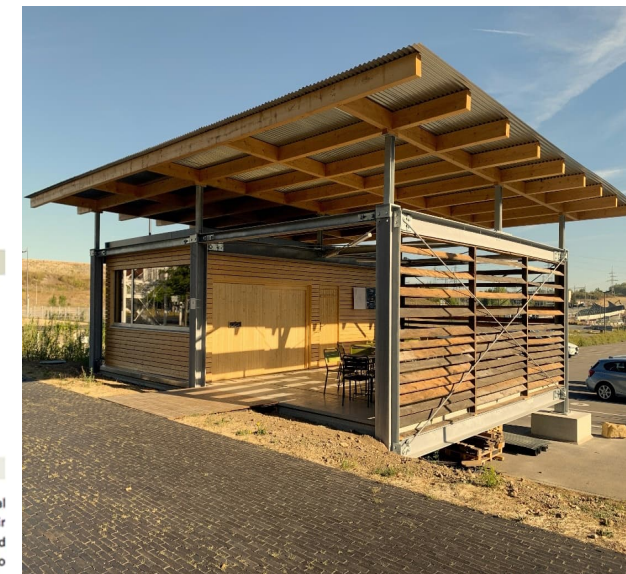
Picture credits: ArcelorMittal
