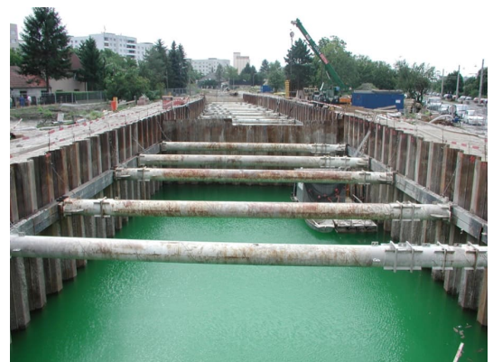
Sheet pile wall with struts
