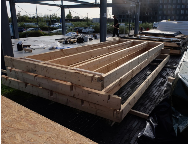
Photo taken during deconstruction © Schroeder & Associés; Timber panels with notches for accessing screw heads during deconstruction.
