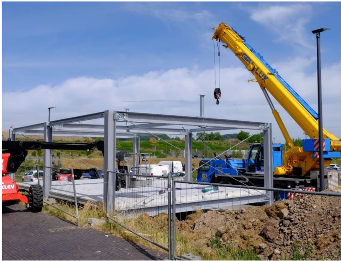
Steel skeleton with prefabricated concrete slabs 1 .
