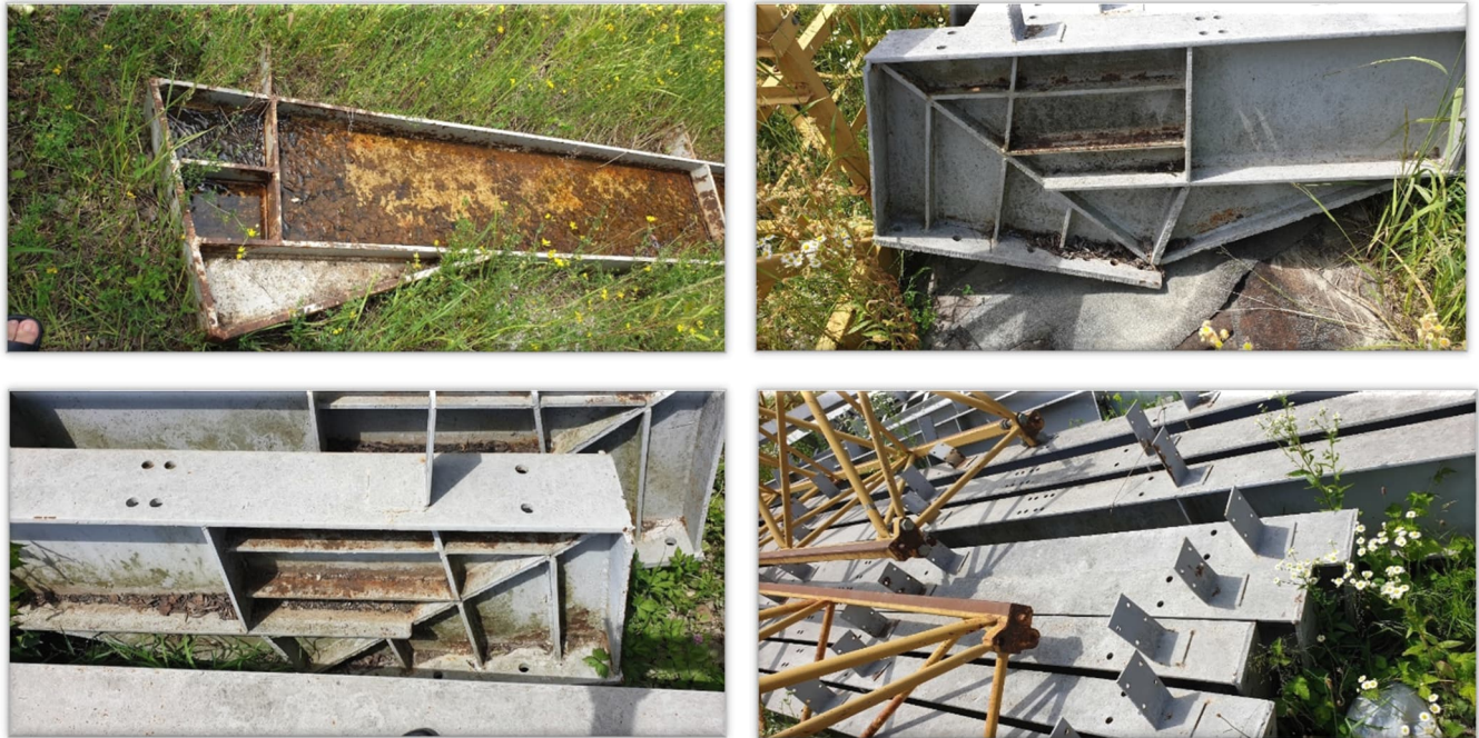
Fig. 2. Components of the existing structures
