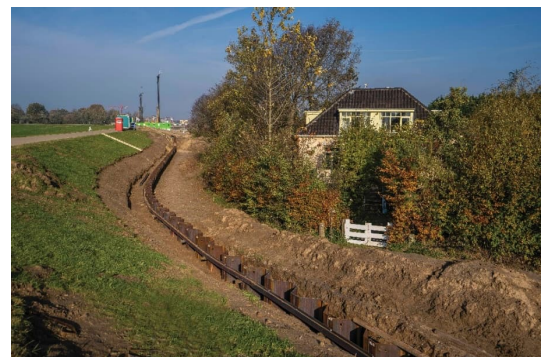
Dyke reinforcement in Wolferen-Sprok NL 2
