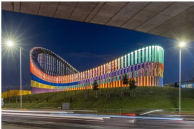
Bent Cross Town Primary Substation, London, UK
