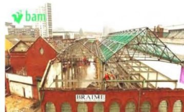
University Technical College, Leeds, UK
