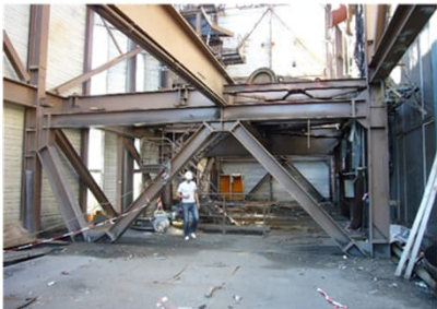
RWTH seminar building, Aachen, Germany
