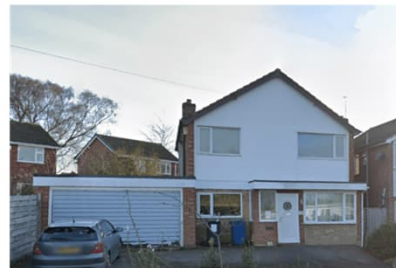
Refurbishment project, Lichfield, UK
